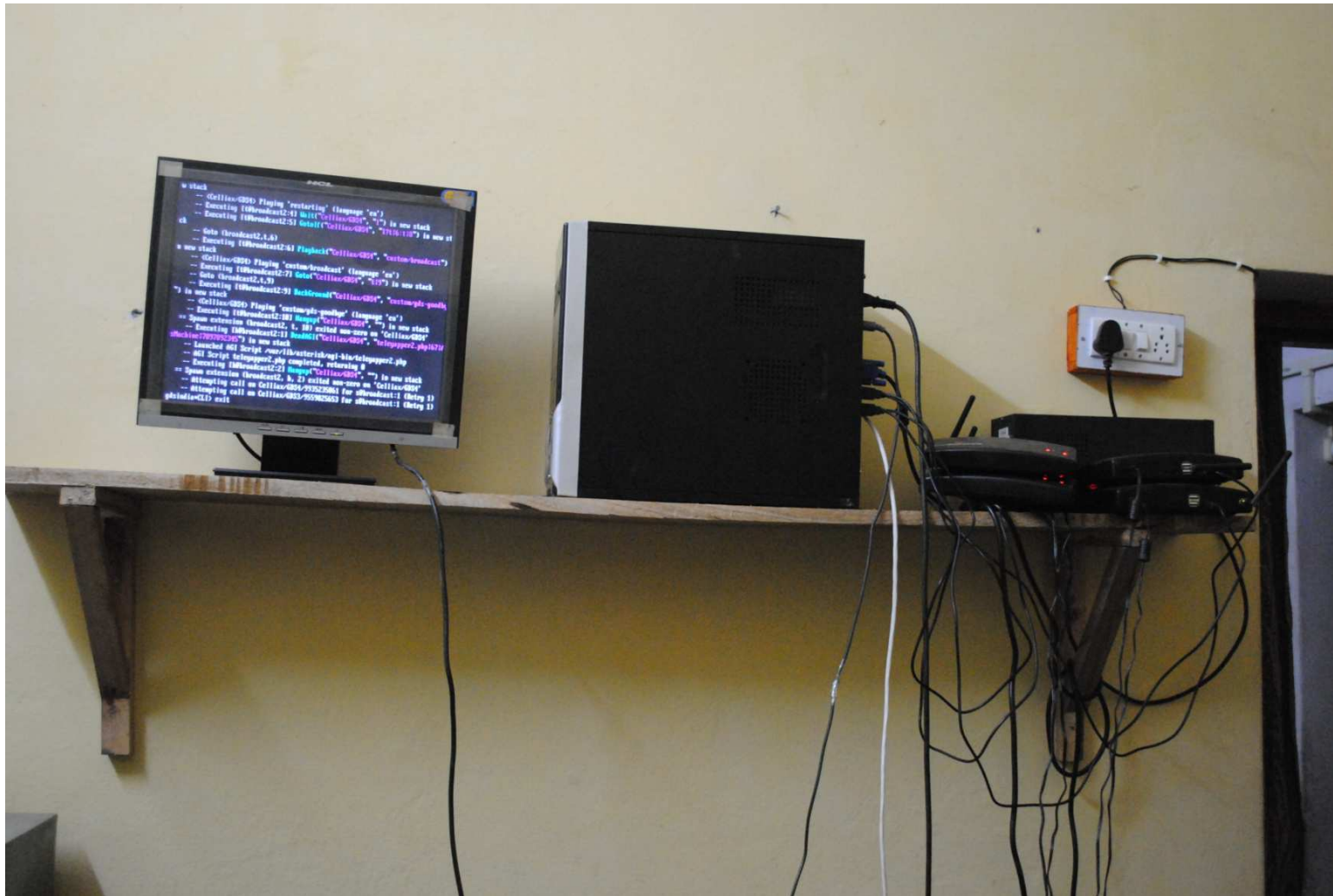
Computer System with Multiple GSM Modems attached
